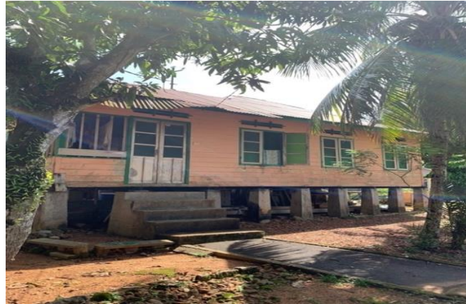
Figure 7. The Original Architecture of the Malay House at Pulau Penyengat
